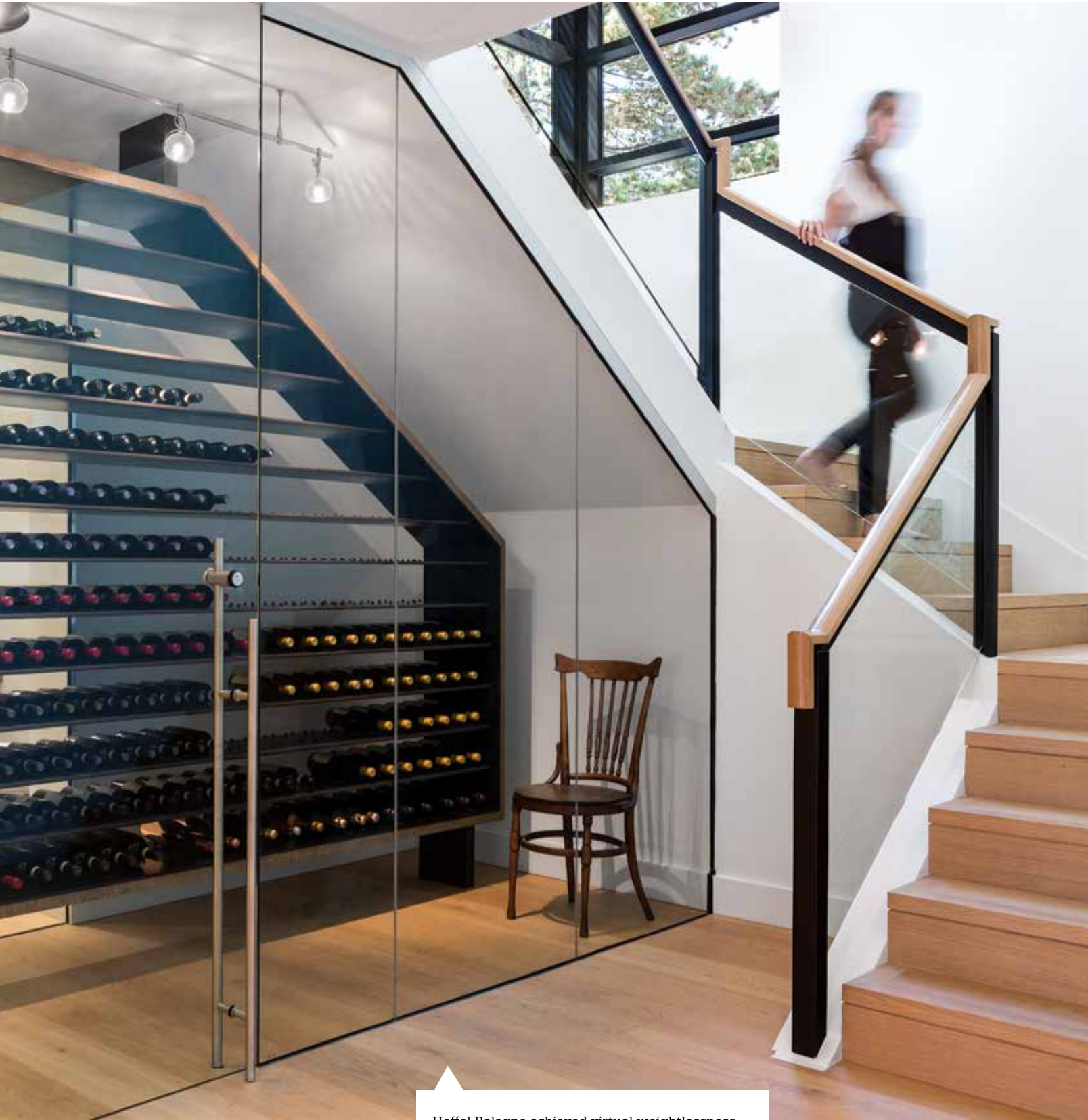
Heffel Balagno achieved virtual weightlessness by floating the wire-brushed oak and burnished steel shelving unit within the space, supporting it by only four thin steel posts.
